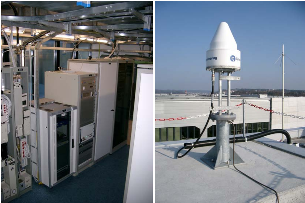
Figure 4.32: Left panel: RIMS and WAN racks at Zurich Airport; right panel: One of the two RIMS antennas.
