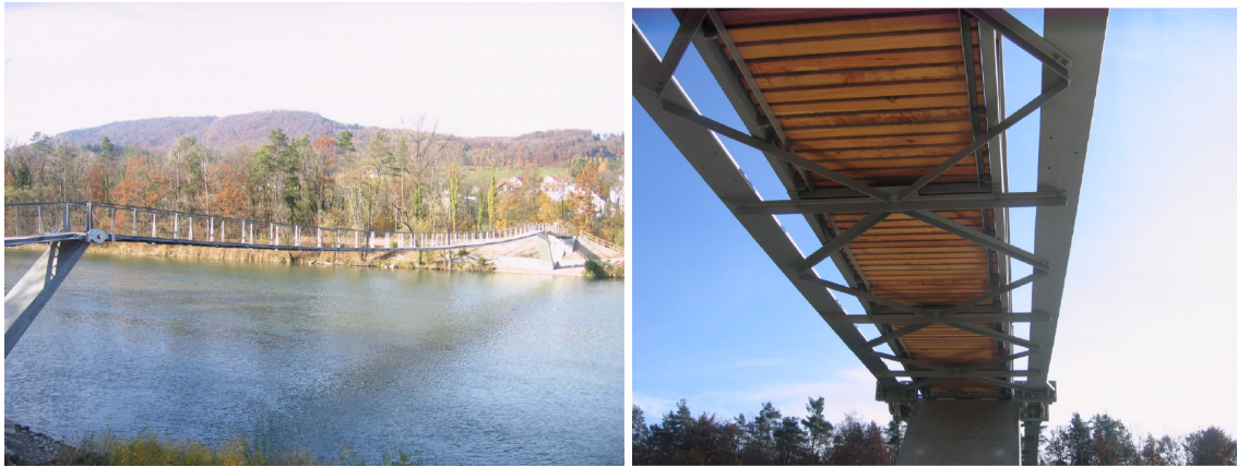
Figure 8.19: The Auen bridge over the Aare river (left). The pedestrian bridge is constructed as a suspension bridge with two longitudinal beams (right).
