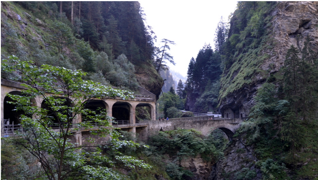
Figure 5.1. Rockfall protection structures and bridges in a 300 m deep gorge (Viamala, Thusis, Switzerland), where the GNSS reception is absent or unreliable for autonomous UAV guidance.
