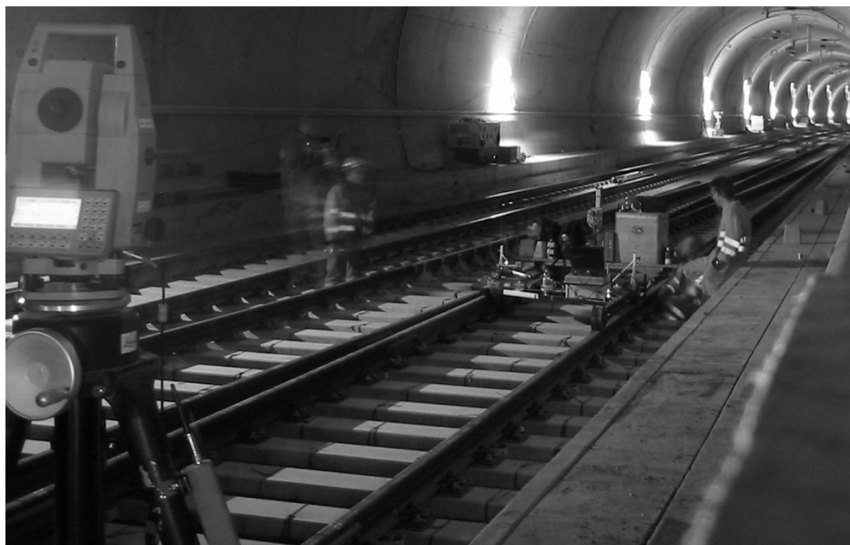
Figure 6-4 TCRA1101 on an industrial tripod used for the coarse alignment in interaction with the Swiss Trolley
